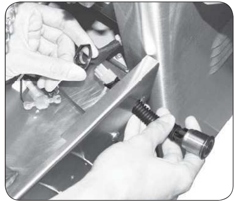
Fig. 2-1 Installing master switch
