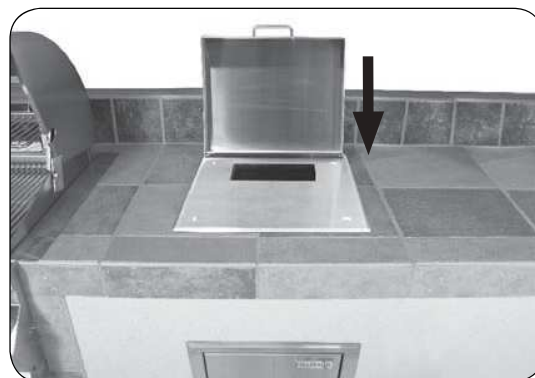
Fig. 3-2 Drop unit into place
